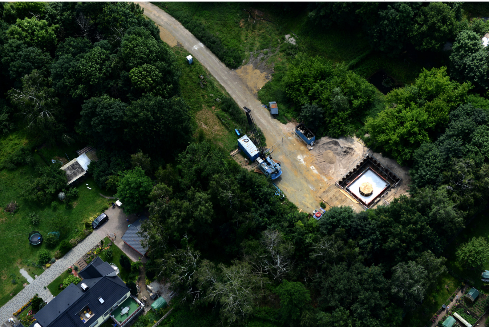
Baugrube des HBr 4 in Senftenberg | P. Radke | 2013
